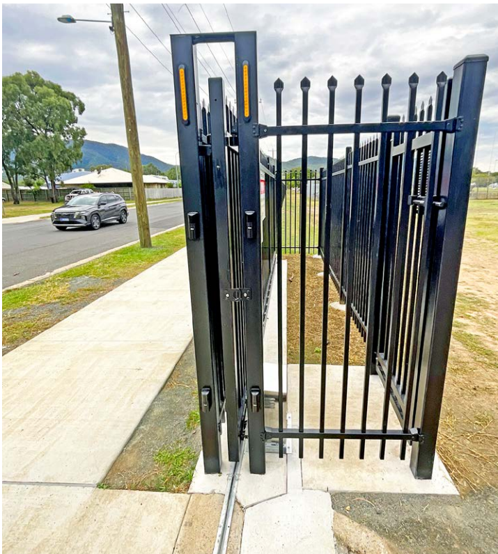
Concrete pad for automated gate motor
